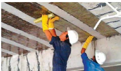
Gambar 6. Pemasangan FRP pada Pelat ("FYFE Company profile," n.d.)
