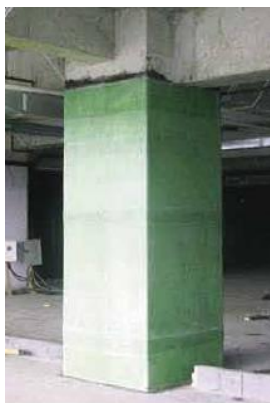
Gambar 5. Peningkatan Kapasitas Kolom Menggunakan FRP ("FYFE Company profile," n.d.)
