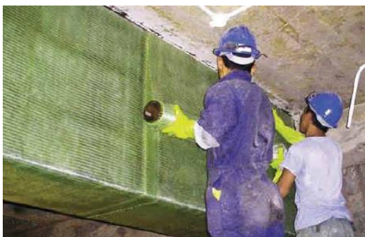
Gambar 4. Pemasangan FRP pada Balok ("FYFE Company profile," n.d.)
