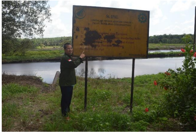
Gambar 6. Instalasi Pengolahan Air Limbah PT. Musirawas Citraharpindo
