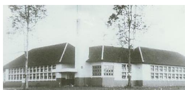
Figure 16: Meanwhile, on beside of the governor office, a streamline architecture or art modern have promoted on the Public Work office covered with white colour, punnet windows and asymmetrical view. (source: Riwut, 2016)
