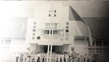
Figure 15: Main entrance of Governor office who still influenced by late type of art-deco style (source: Toemon, 2018)
