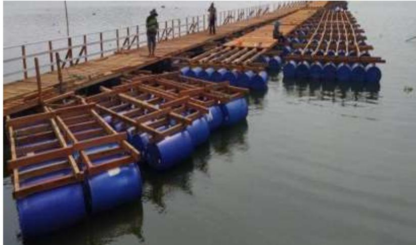
**Figure 1** Plastic Drum Platform Material [4]
